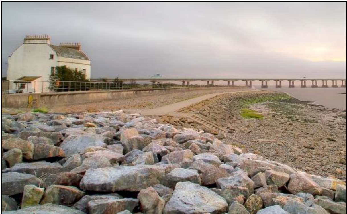
Picture 1 – M4 Prince of Wales Bridge looking south from New Passage
