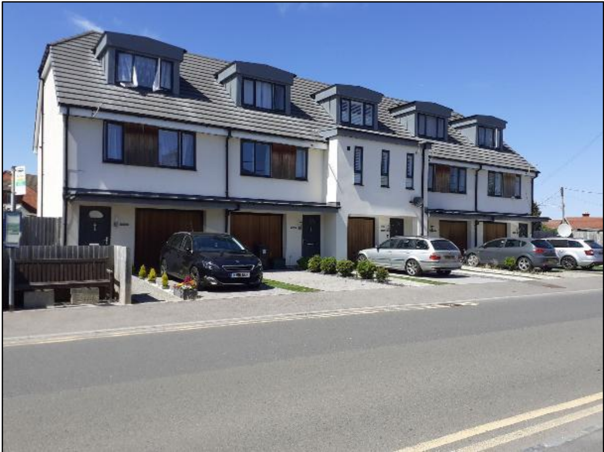
Picture 12 – New housing in Severn Beach designed with flood mitigation.
