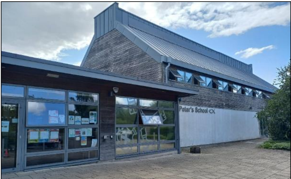
Picture 6 – St Peter's Primary School on Bank Road, Pilning
