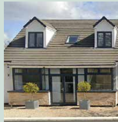
Figure 132: - Porch, provides passive heating (Trombe Wall).
