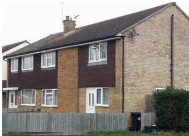
Figure 59: - Part non-cavity constructed dwelling.
