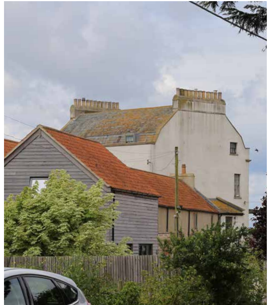
Figure 109: - Red clay tiles with complimentary facade materials.
