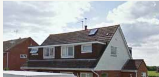
Figure 102: -Flat roof dormers, reduced performance and space.
