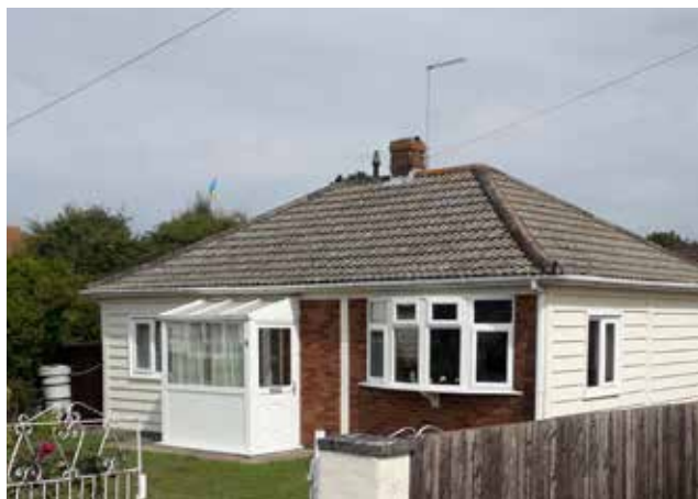
Figure 58: - Concrete panel construction, Victoria Crescent.
