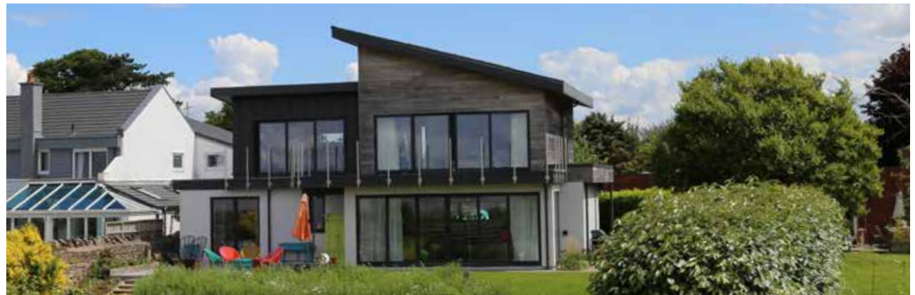
Figure 32: - Composition of flat and monopitched roofs and facades in render, standing seam and composite cladding. generous window openings
