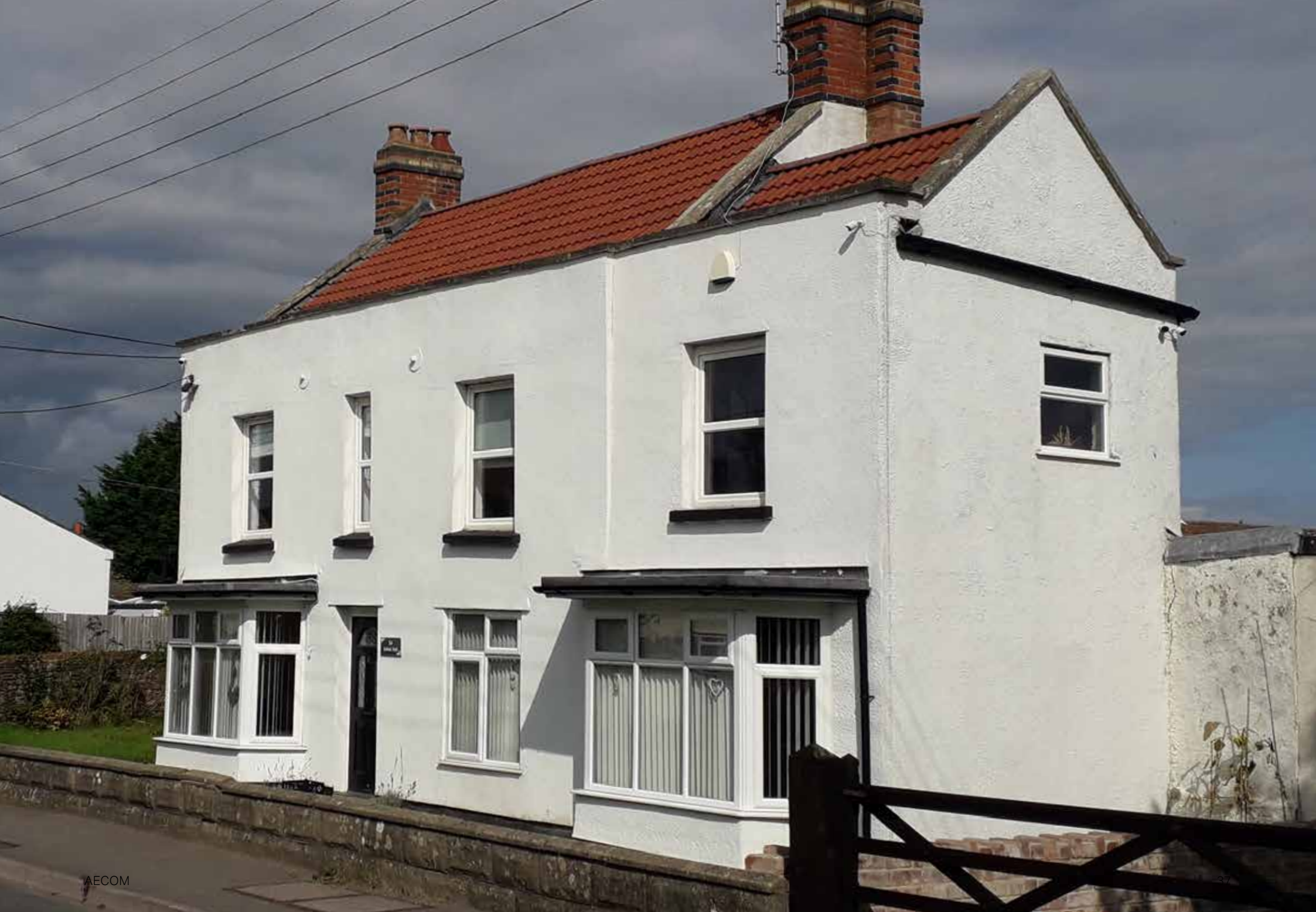
Figure 23: - Parapet roof rendered property with decorative brick stacks.
