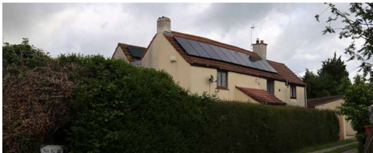
Figure 26: - Pitched property with potentially problematic large flat roof valley and twin PV array.
