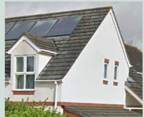
Figure 133: - Thermodynamic panels, Ashley Court.
